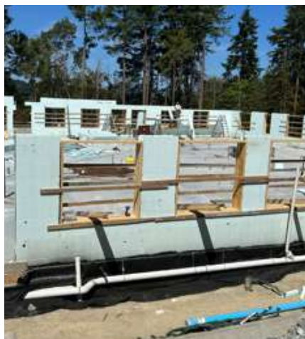
Window openings framed
